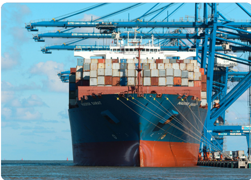
Steep mooring-line angles on larger vessels reduce horizontal restraint and increase bollard uplift. Berths designed for smaller vessels may need revised mooring arrangements.
