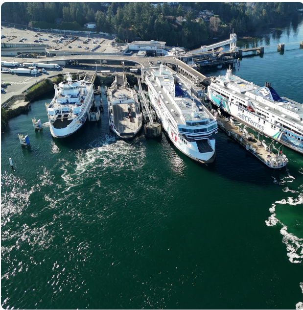
Our BC Ferries terminal work covers floating wing walls, dolphin and berthing loads, and storm tie-up mooring analysis.
